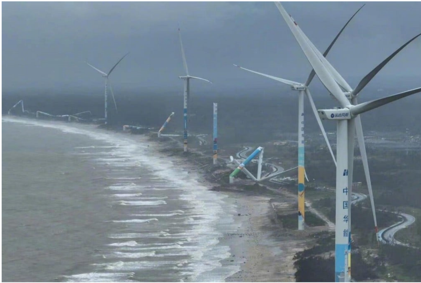
Wind turbines damaged by Typhoon Yagi (Sept. 2024)
